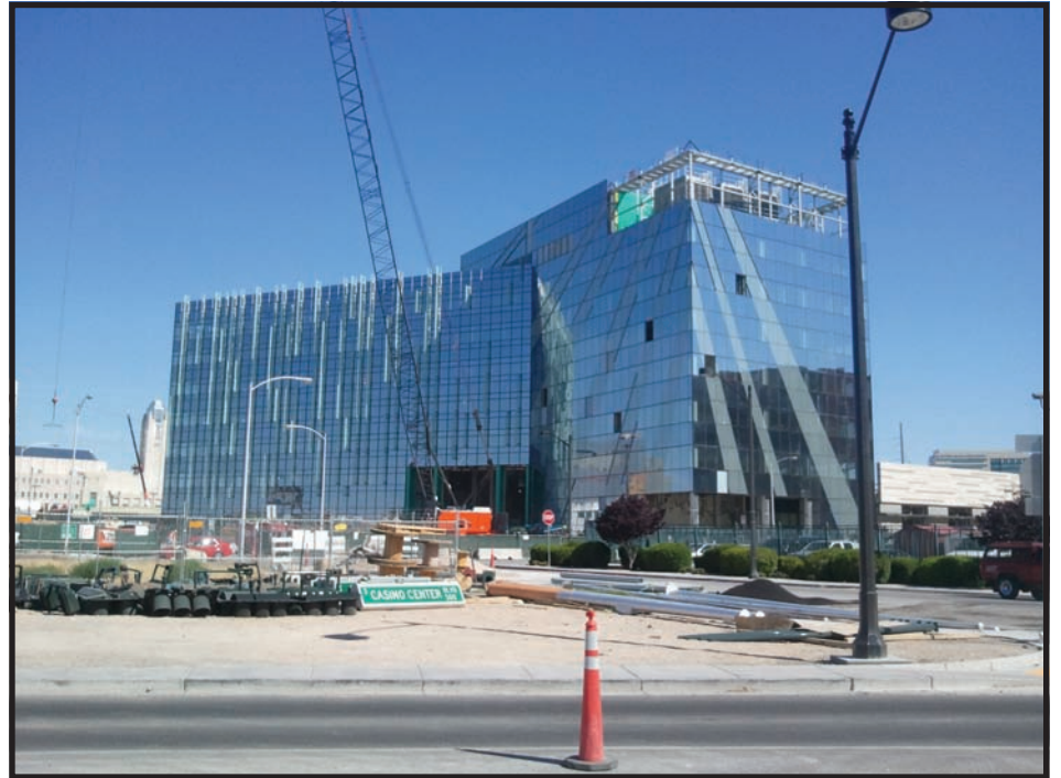
The new City Hall nears completion
