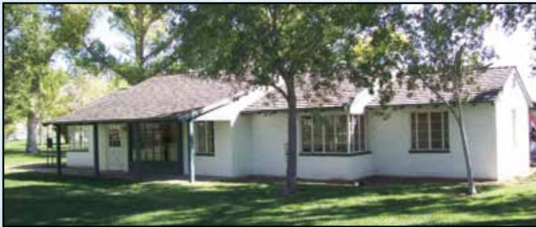
Foreman's House, Floyd Lamb Park at Tule Springs
